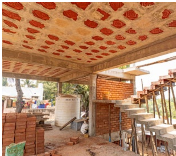
Building site : work in progress
