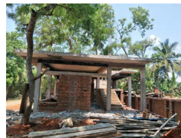
The Construction Site - July 2020
