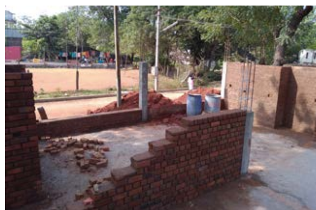
The First Steps of Construction
