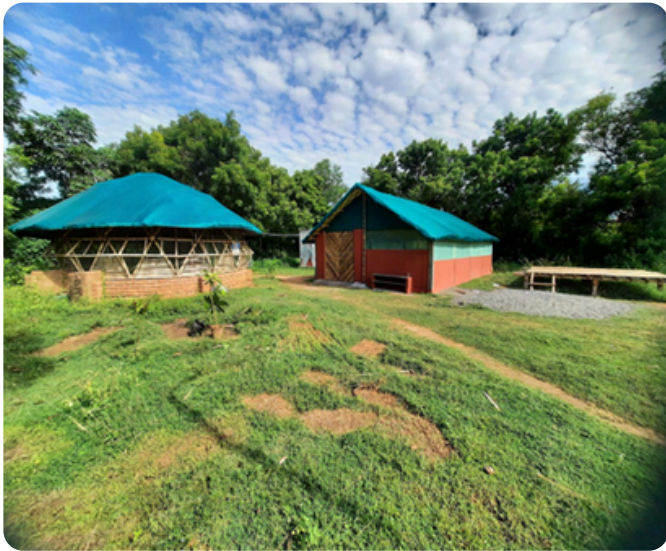
The bamboo structure in Edayanchavdi after-school
